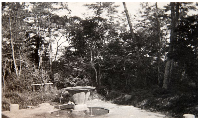
Nara, Tōshōdaiji, ornamental water vessel.
